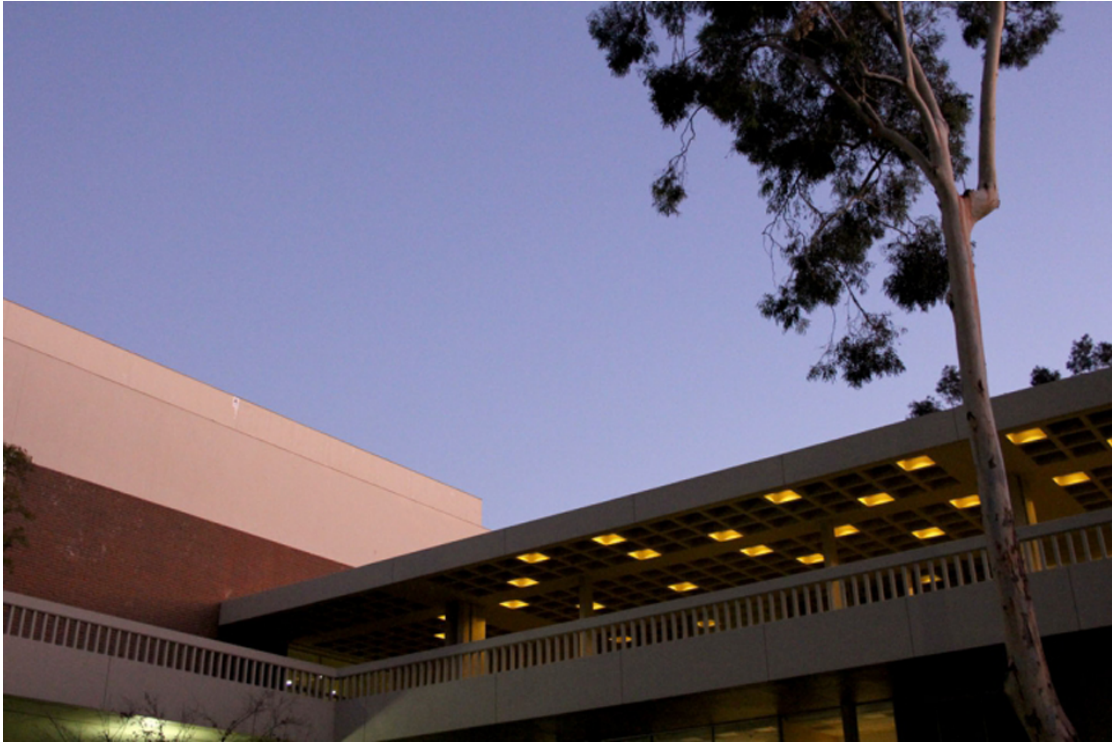
FIGURE 5.2: A distance view of the waffle-ceiling above the main entrance with an assortment of fluorescent lights
